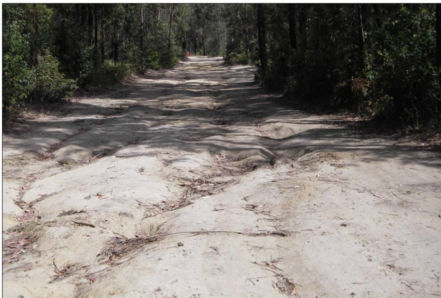
Plate 3. Road within the Estate.
