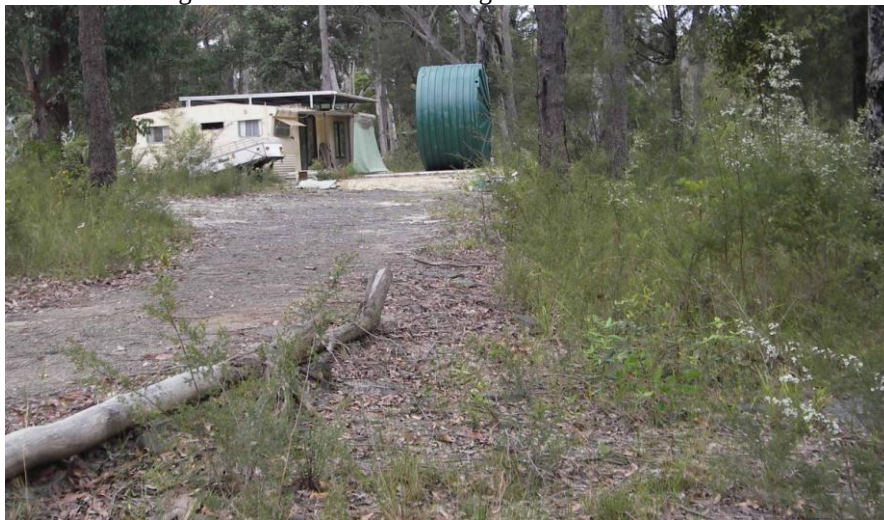
Plate 2 Minor structure on Lot 145 Greenslopes Avenue
